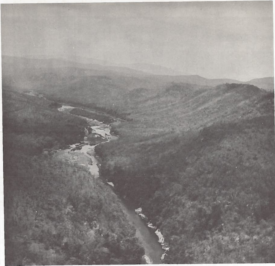
Figure V-53--Lower Diddessa damsite (DD-2), looking upstream. The dam, 320-mw. powerplant, and transmission facilities will be the major features of this single-purpose hydroelectric power project.
