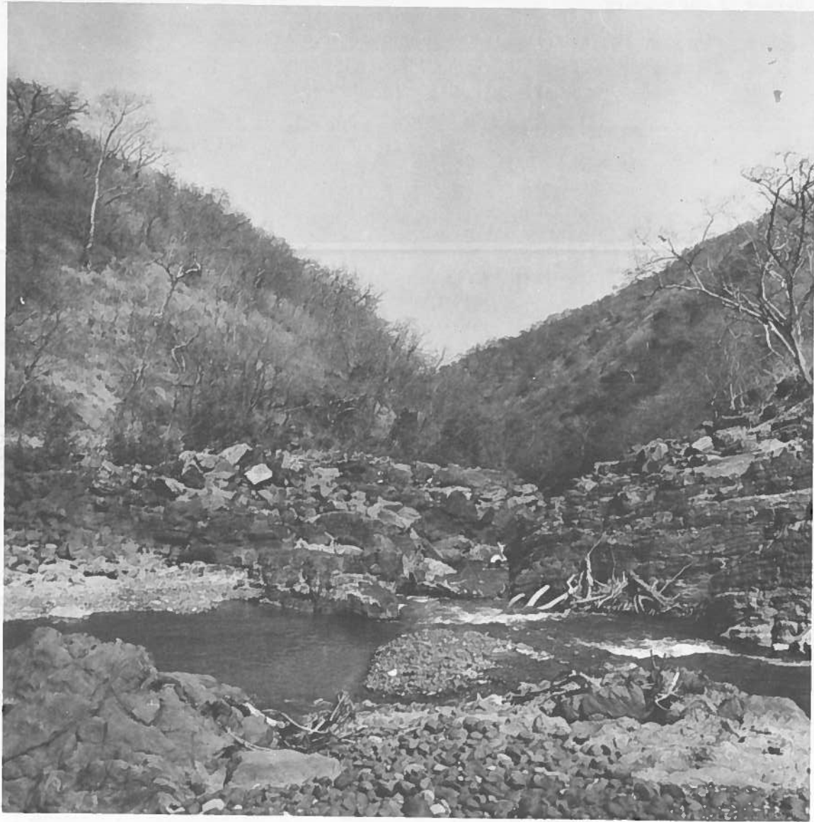
Figure V-51--Lower Guder Project damsite (GU-1) looking upstream. The dam, 50-mw. powerplant, and transmission facilities will be the major features of this single-purpose hydroelectric power project.
