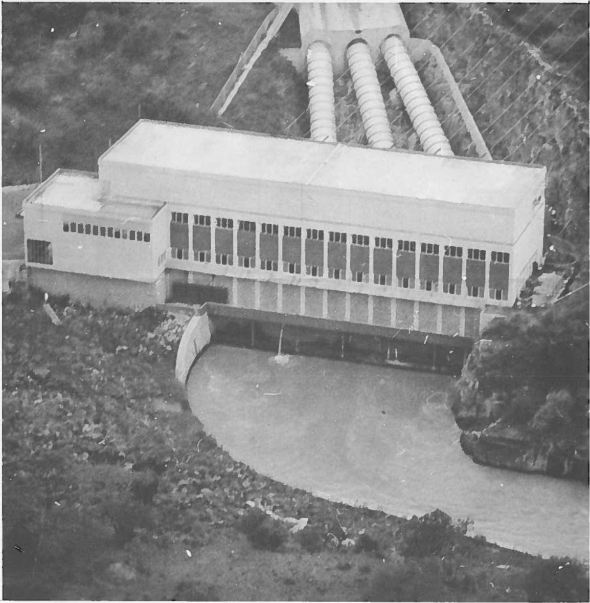
Figure V-21--Koka hydroelectric powerplant utilizes a head of 32 to 40 meters and has three generating units, each rated 18,000 kv. -a. It has a firm generating capability of about 23,000 kw.
